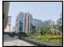
External View of Subject Property
