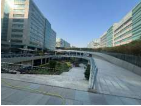
External View of Subject Property
