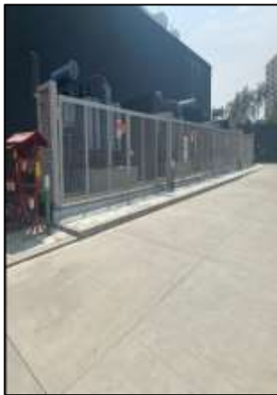
View of Power Back-Up
