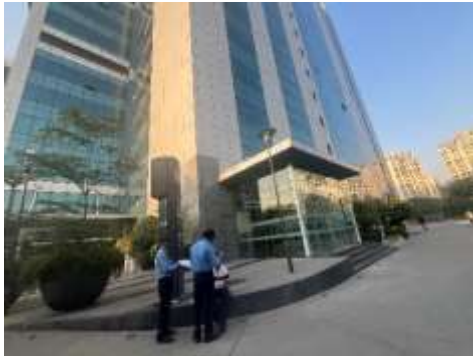
External View of Subject Property
