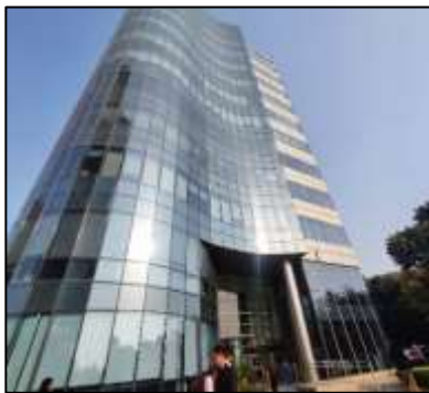
View of Block 1
