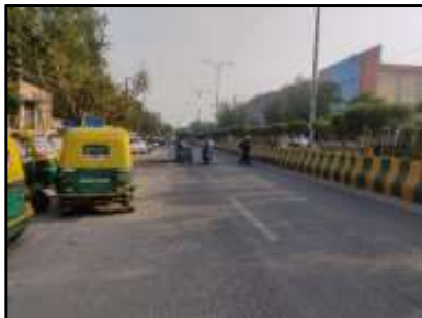
View of Access Road
