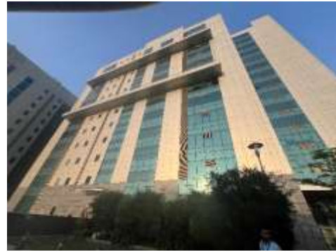
External View of Subject Property
