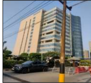
View of Block 2
