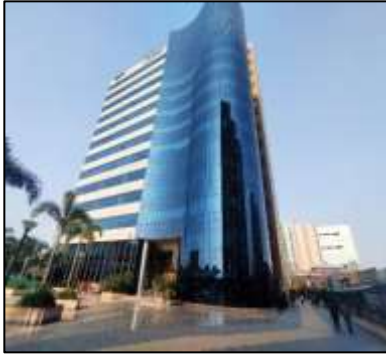
View of Block 3
