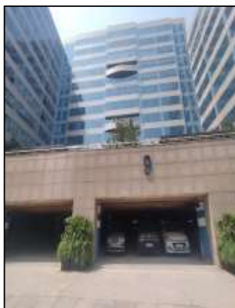
View of Tower 9
