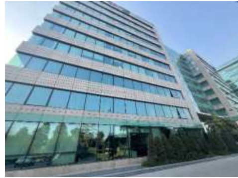
External View of Subject Property
