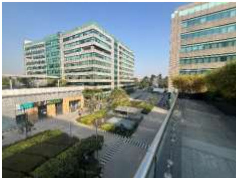
External View of Subject Property
