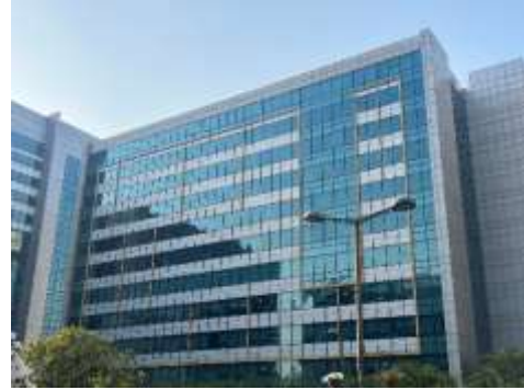
External View of Subject Property
