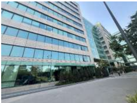
External View of Subject Property
