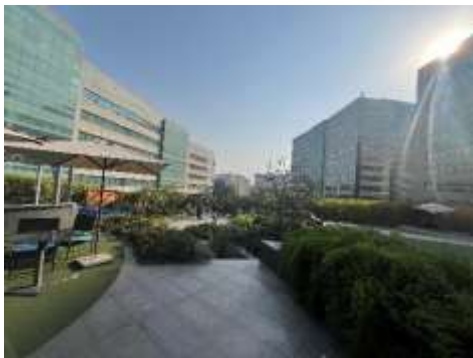
External View of Subject Property
