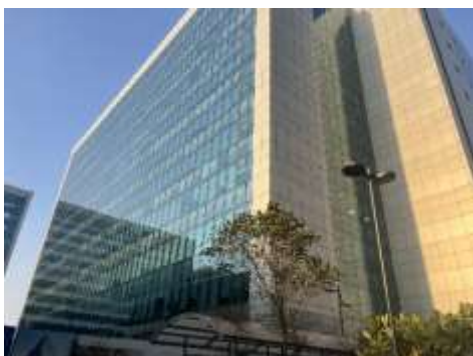
External View of Subject Property
