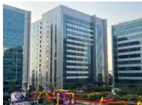
External View of Subject Property
