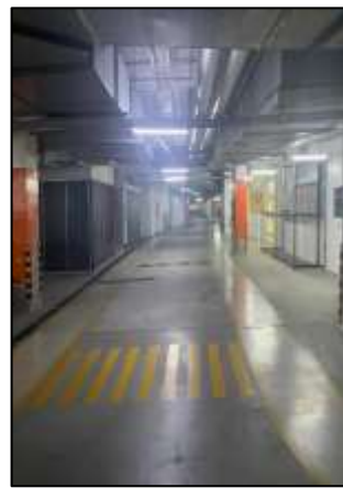
Internal view of Tower 6
