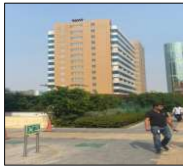
View of Block 6
