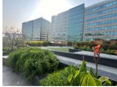
External View of Subject Property
