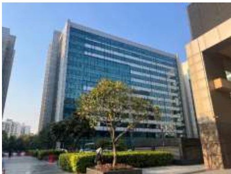
External View of Subject Property
