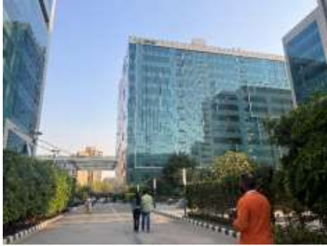
External View of Subject Property
