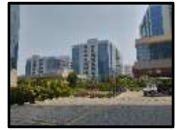
External View of Subject Property
