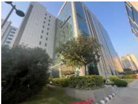
External View of Subject Property
