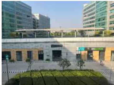
External View of Subject Property
