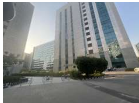
External View of Subject Property
