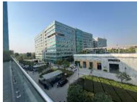
External View of Subject Property
